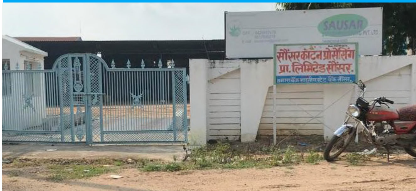
Picture 5: A locked health centre in Chhindwara District
