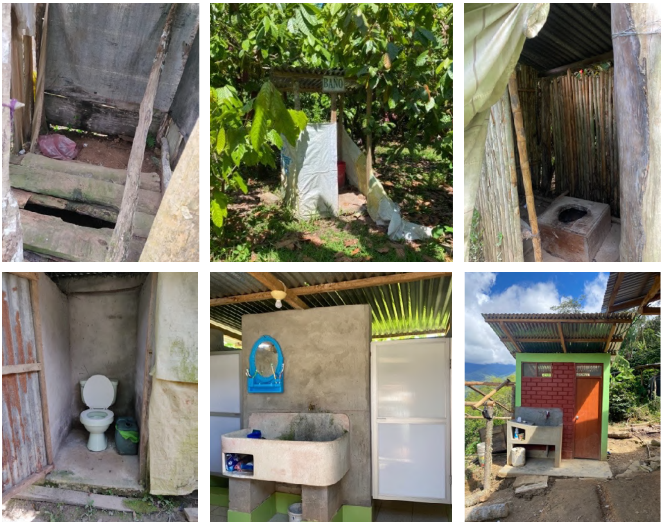
Notes: The first row of pictures shows several cesspits, all located in the backyard of the houses. The second row shows toilet facilities constructed with brick and cement. The last picture is a toilet facility constructed by a community project in Cajamarca. Sources: Authors' photos.
